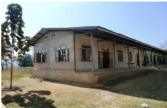
New school building construction (50x30) feet Expenditure - 5,455,420 MMK
