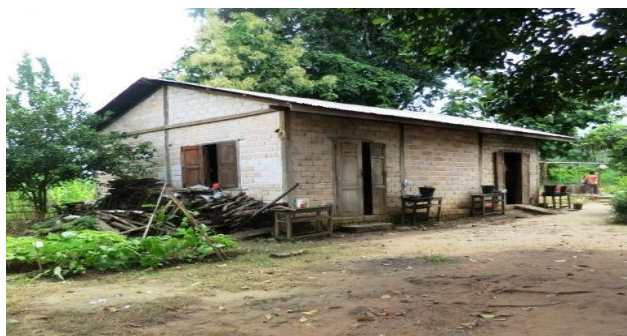
Teachers accommodation construction expenditure - 553,300 MMK
