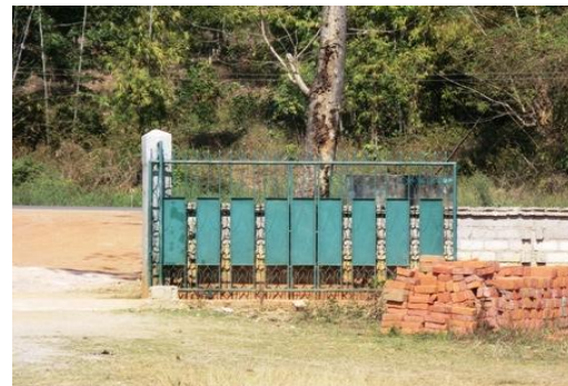
School compound fence and gate construction Expenditure - 1,625,500 MMK
