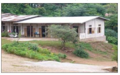
started to build extension and completed its foundation and frame with a part of zinc roofing about 3 years ago. But it had been suspended due to lack of fund. The new school building is 40 x 30 feet size, block nogging walls, zinc roofing, concrete floor, 4 doors and 6 windows.
